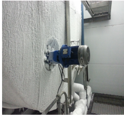
Side-entry mixer on a 50 000L horizontal cold-stabilisation tank, running at - 4C
