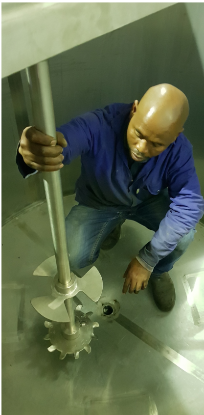
Installing a top entry fruit lagoon mixer
