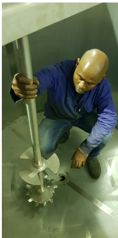
installing a top entry fruit lagoon mixer
